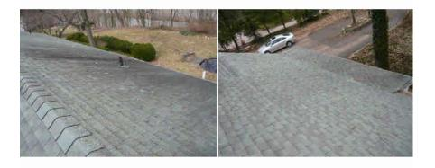
Estimated age of roof covering: 5 - 7 Years. Dimensional shingles (Timberline Architectural Shingles) have 25 to 30 year average life span. General condition appears serviceable with signs of weathering and aging. Regular maintenance and inspections are advised.
