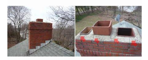
Chimney Flashing: The chimney flashing appears satisfactory. **Repair or replace the concrete chimney crown to prevent moisture intrusion and chimney damage**. Chimney cap is recommended. Flue Liner: Visible. Hire chimney sweep to evaluate & clean flue - The flue should be cleaned for safety prior to closing. The internal elements of the chimney fall
