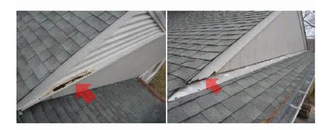
**Rot or deteriorated material** - Recommend replacing all defective areas at this time to protect the surface behind the trim. Soffit: The soffit is in satisfactory condition as is. Soffit is vented. Facia: The visible facia is in satisfactory condition.
