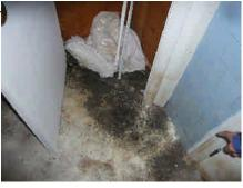
WALLS & CEILING: Tile. Loose and missing tiles are viewed at the wall. Repair.
