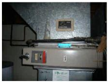
and dirt in the blower section. Have the filter inspected by professional. You could have a blocked cooling coil and that will reduce your heating and cooling. Humidifiers are not fully inspected in this home inspection reports and are beyond the scope of standard set by the state of New Jersey.
